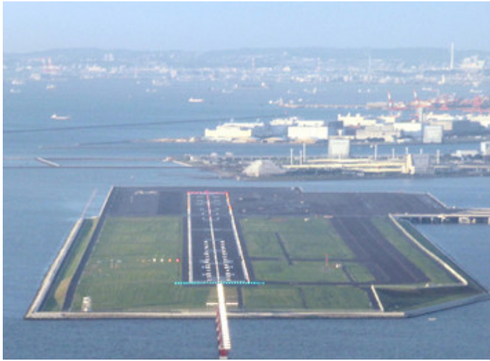
Figure 2. Aerial Photo of D-runway, as of the 29th of September, 2010
